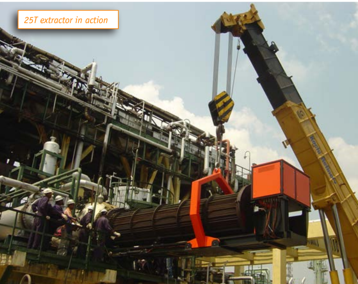
45T bundle puller with 2 meter rear extension (6.5 feet). Pulling 10 meter bundle (33 feet)
